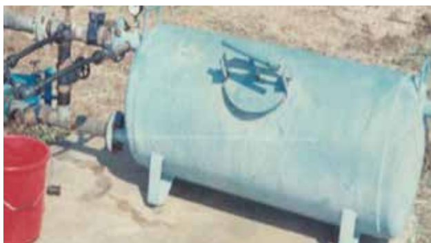
Fig. 8: Fertigation with Venturi
